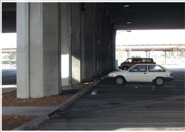
Figure 4: Parking Lot in Wilmington Station
