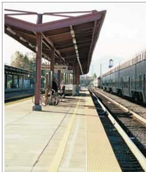
Figure 2 – Caltrain San Jose station Source: http://www.capitalcorridor.org/
